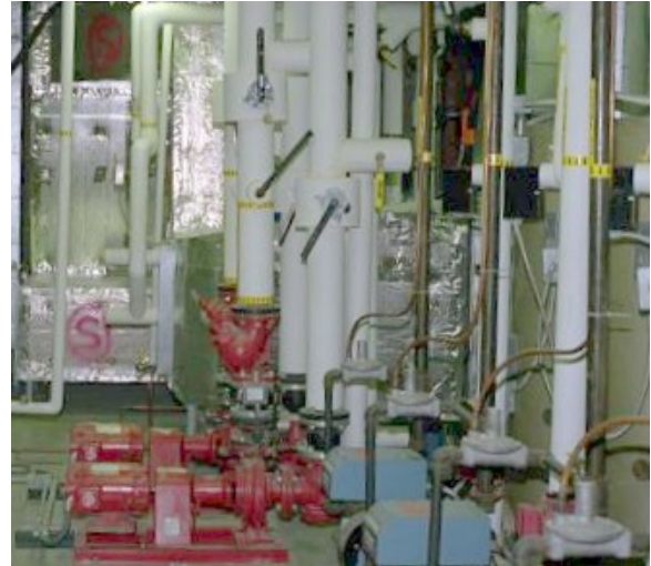
Figure 159—Loop Water Pumps and Piping
