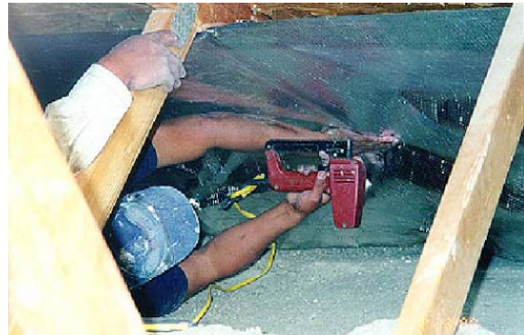
Figure 113—Installing Radiant Barrier
