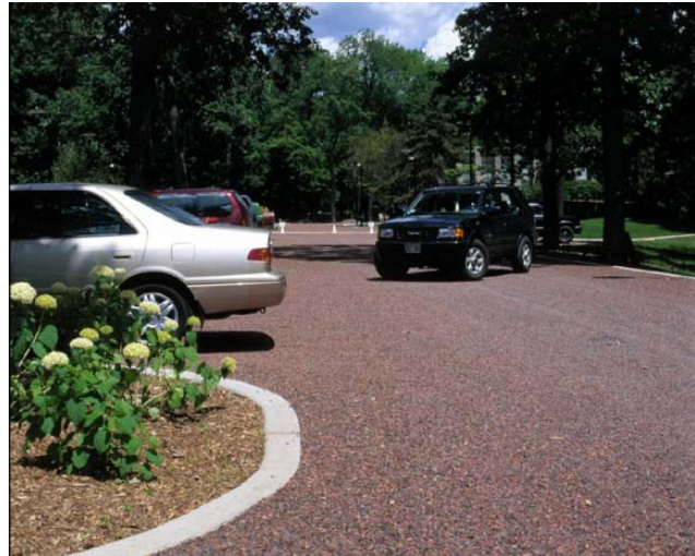
Figure 16—Porous Parking Lot
