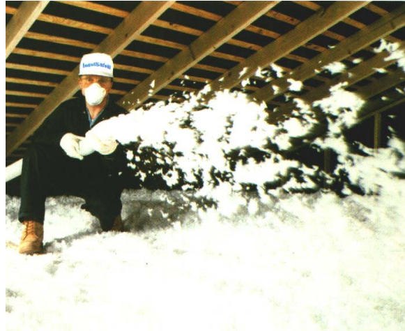
Figure 109—Blown-In Insulation
