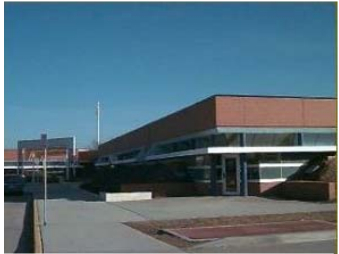
Figure 65—Exterior Light Shelves
