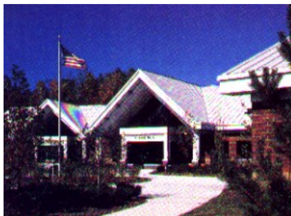
Figure 111—Standing Seam Metal Roof with White Coating
