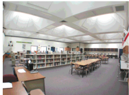
Figure 44—Deeply Coffered Ceiling
