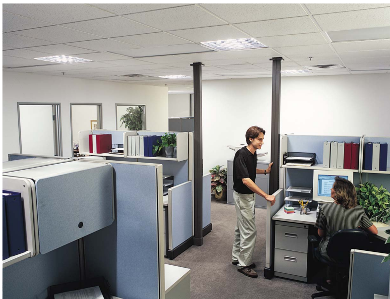
Figure 75—Tubular Skylights in Interior Office
