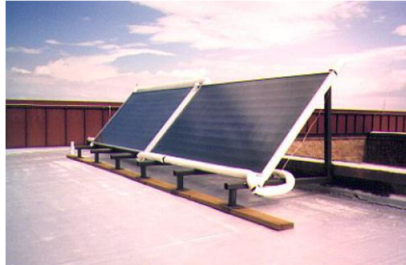
Figure 160—Solar Hot Water Panels
