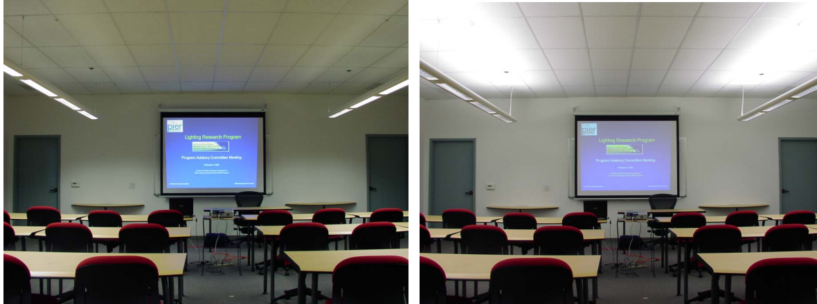
Figure 82—Dual Mode Classroom Lighting System
