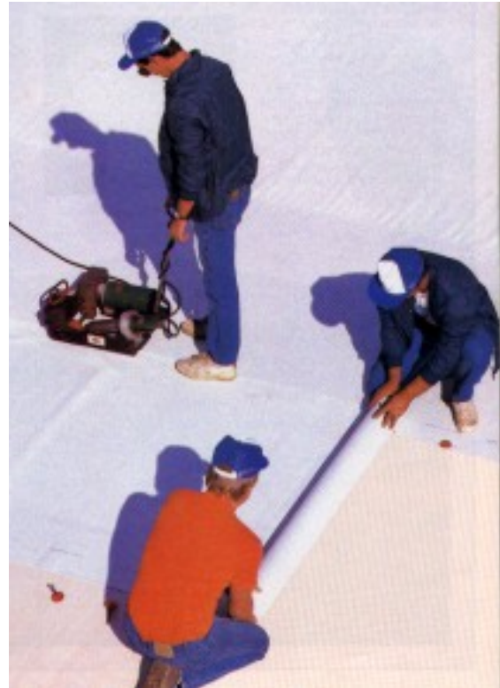
Figure 110—White Single Ply Membrane with Heat-Welded Seams
