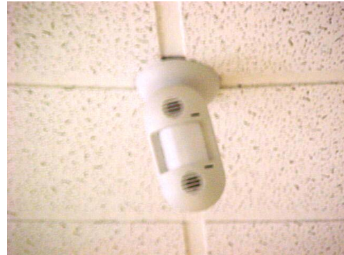
Figure 88—Ceiling Mounted Photosensor
