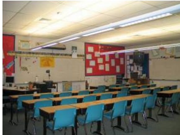
Figure 78—Indirect/Direct Lighting System
