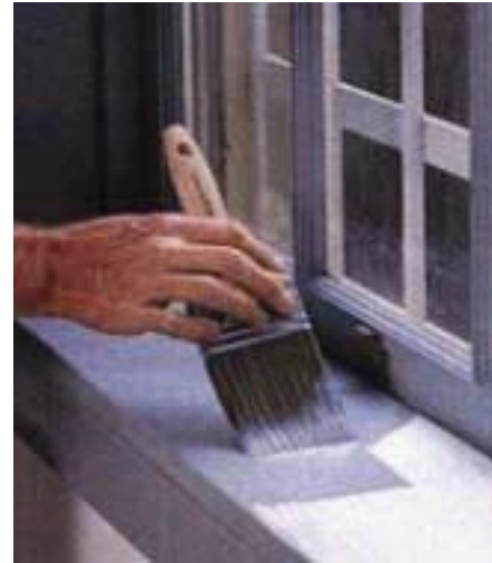
Figure 35—Paint Being Applied
