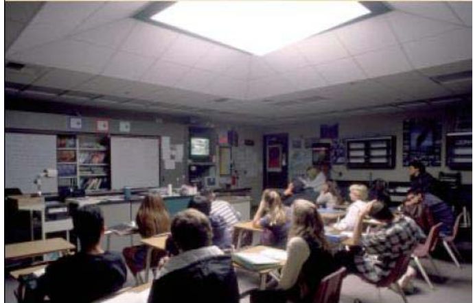
Figure 119—Skylight Used at Capistrano Unified with Dimming Controls
