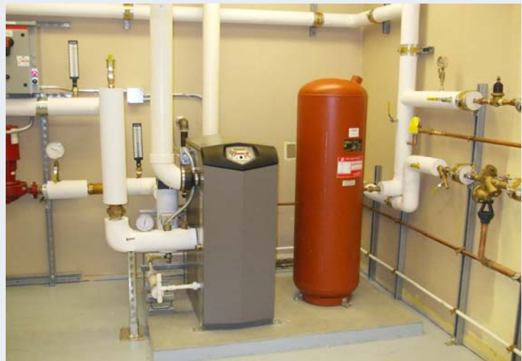
Compact Condensing Boiler Installation
