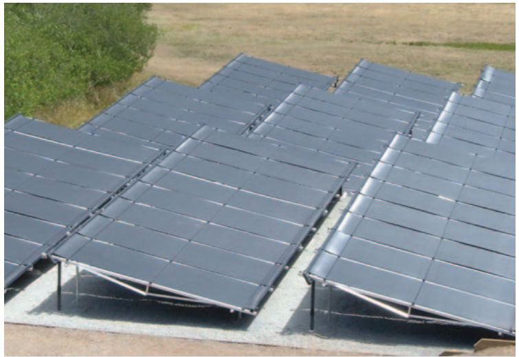
Fig. 12. FAFCO commercial system collector array in California. Photo from FAFCO
