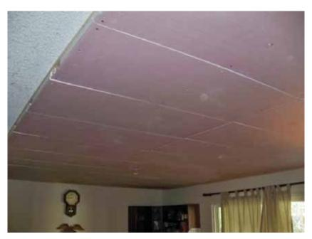
Figure 39: Uponor Panels Installed In the Grandstaff House (Prior To Finishing)
