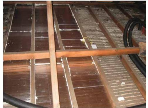
Figure 88: Foil Faced Foam Insulation below Wiring
