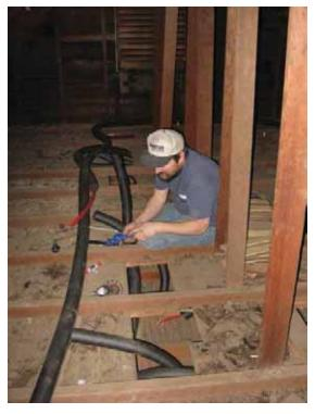
Figure 45: Radiant Panels Installed In the 6th Avenue House
