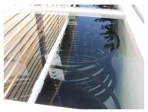
Figure 19: Storage Tank with Evaporator and Heat Exchanger Coil
