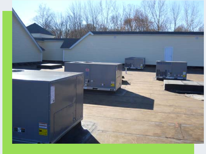
Screened Rooftop Units
