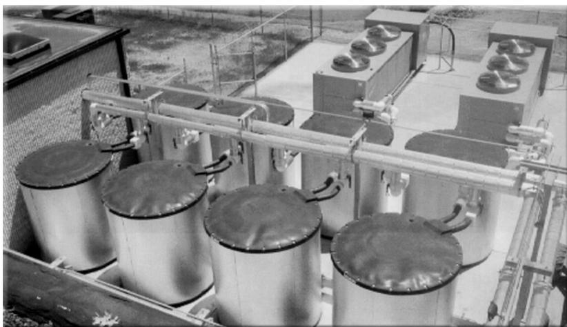
*Modular ice-on-coil storage tanks with condenser units above*
